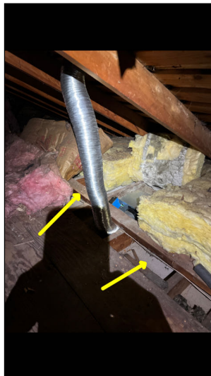
Areas an attic or sparsely insulated.
