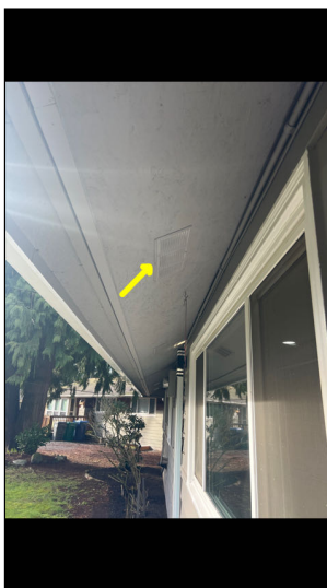
Under eave soffit inlet vents noted.
