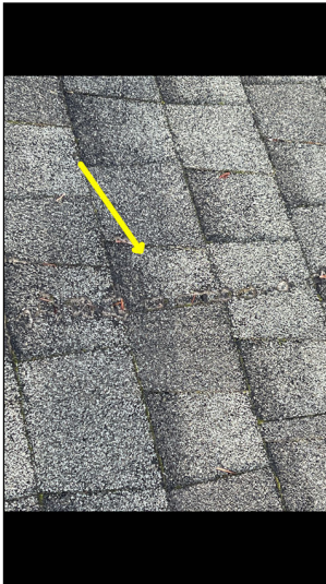
Damaged shingles.
