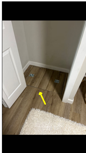
Crawl space access
